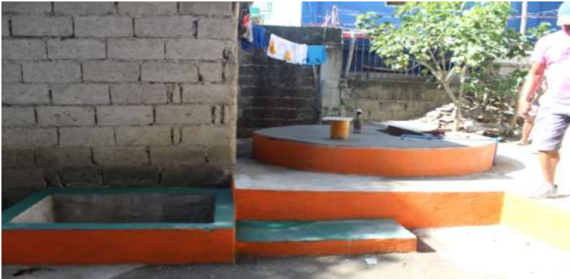
20 Cubic Meters Fixed Type Biogas Digester of Brgy. Gregoria de Jesus, GMA Cavite installed under the technical supervision of Mr. Templonuevo
